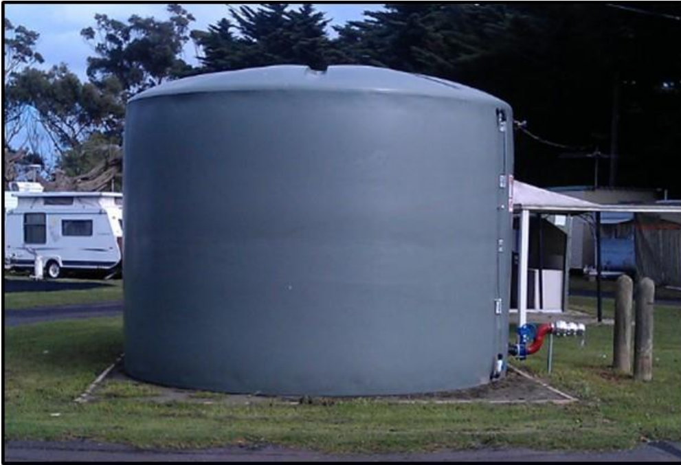
Figure 22 – Example of static water tank supply with Storz couplings
